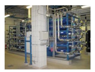
The reverse osmosis system in the large lignite-fired power plant Lippendorf nearby Leipzig, Germany, produces up to 1,200 cubic metres of water for the water-steam cycle every day.
